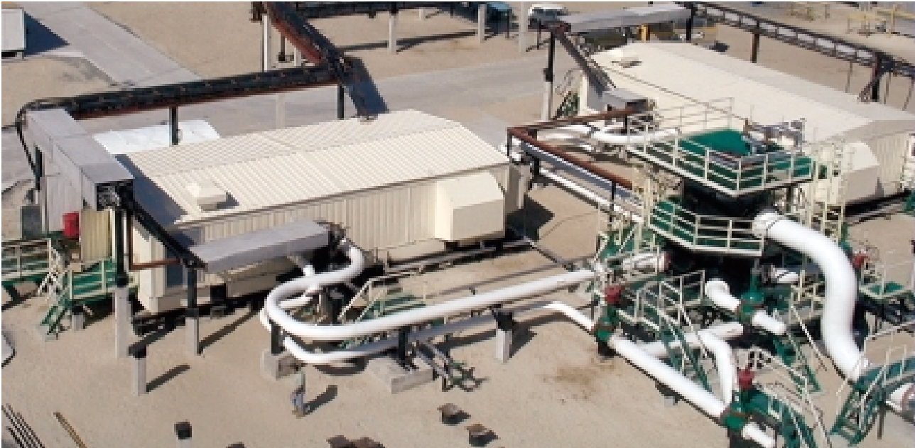
The two multiphase pump shelters installed on site in Siberia
