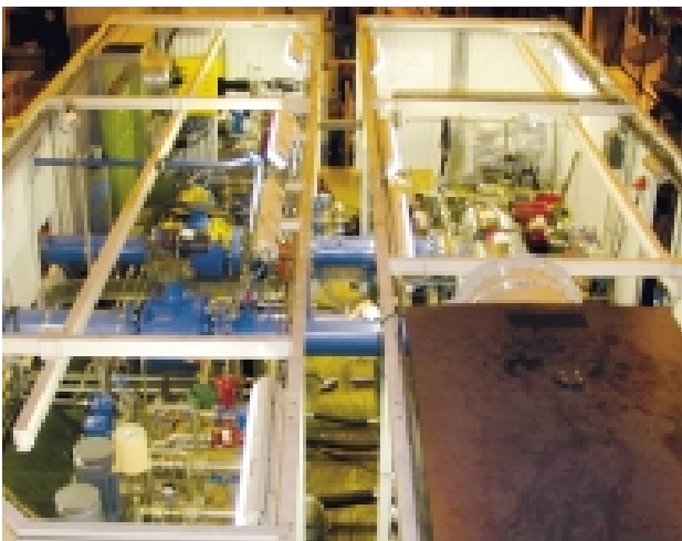
Internal View of Pump Shelter
