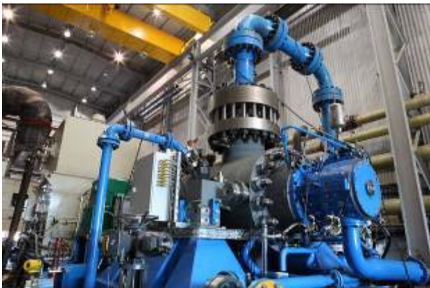
Sulzer boiler feed pump being tested before delivery.
