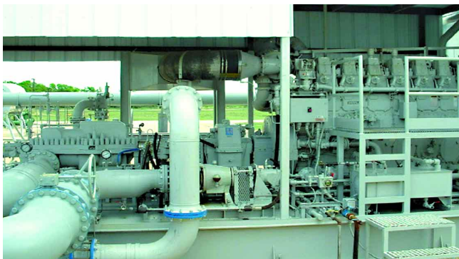
(Left and right) 100K BPD PW Injection Pump and Booster
