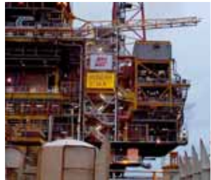
MPP module added to side of existing platform.
