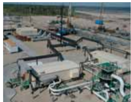
Phased installation: two MPP sets installed.
