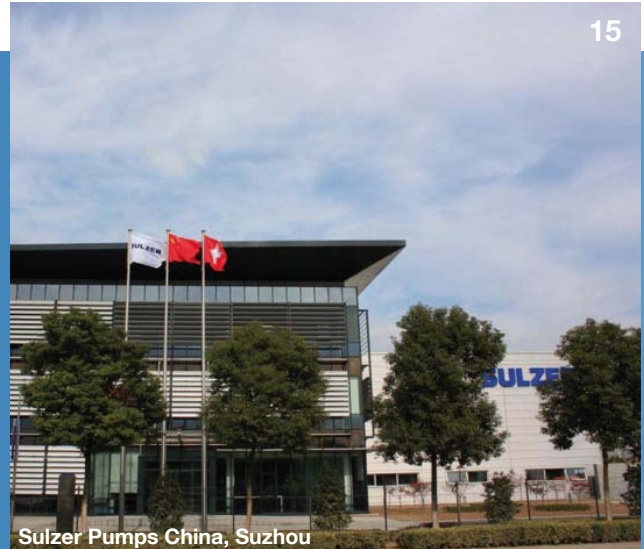
Sulzer Pumps China, Suzhou
