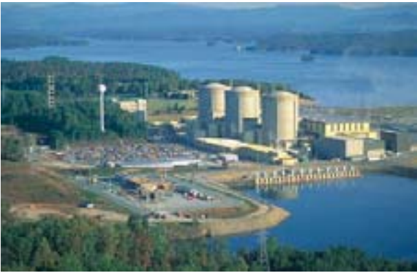
1 Duke Power has awarded Sulzer Pumps a contract to repair and upgrade to nuclear-safety standards twelve cooling water pumps for the Oconee Nuclear Station in the USA.
